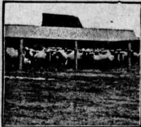
Adequate Protection From North and West Storms in Winter Is Afforded by This Inexpensive Open Shed, Which Faces East.
