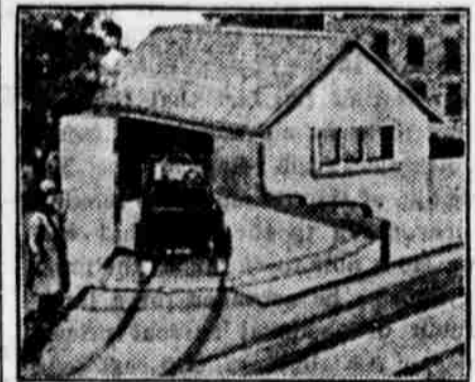
This Side Door, to Which a Low Platform Supported by Wheels is Attached, Makes a Garage Facing on a Narrow Alley Easily Accessible.
