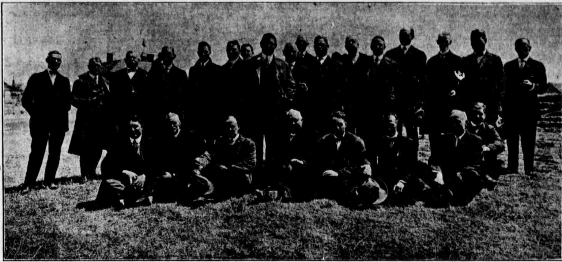
GROUP OF WELL KNOWN MEN PRESENT AT BREAKING OF GROUND IN SOUTH OMAHA ON FRIDAY FOR THE NEW SKINNER PACKING COMPANY PLANT
