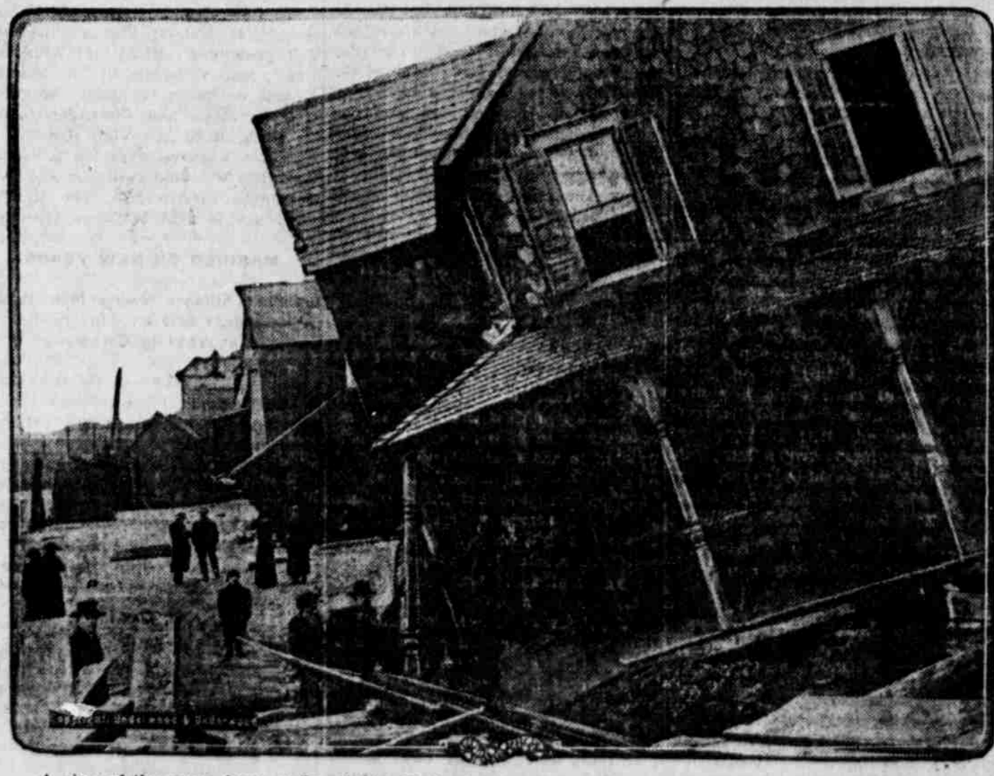
A view of the ocean front at Sea Bright, N. J., showing the wreckage left in the wake of the angry sea, which was lashed into a fury by a 95-mile hurricane that almost destroyed this summer resort on the Jersey coast. Enormous damage was caused by the undermining of the foundations of residences, which resulted in the almost complete destruction of the homes, sending hundreds fleeing into the streets, poorly clad to withstand the biting winds.
