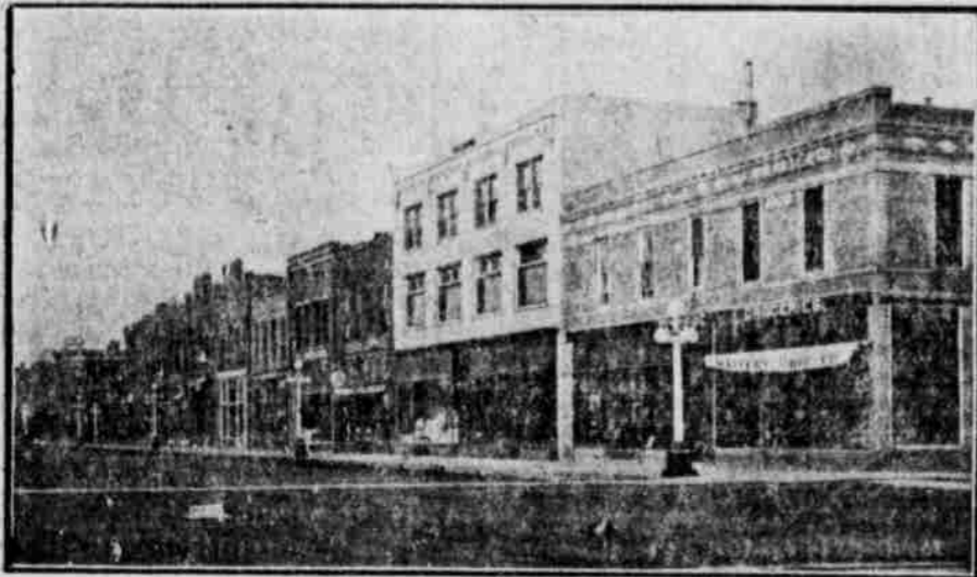
LOOKING SOUTH FROM MALLERY CORNER
