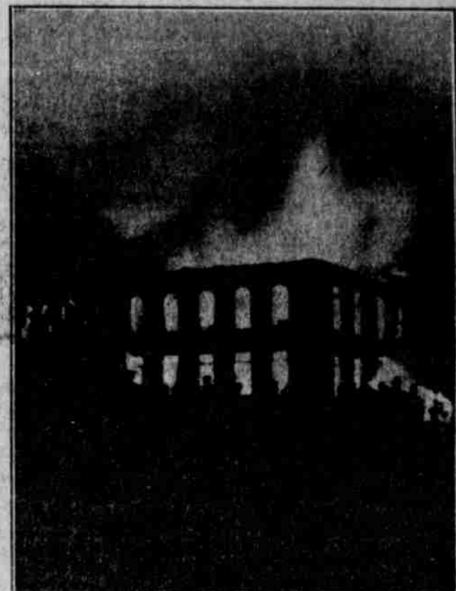
Fire, after roof had fallen, south-east corner of building. Photo by Ben Anderson.
