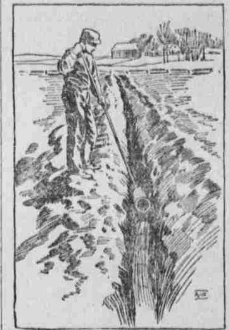
FIG. 11—POOR WAY TO LAY TILE.
