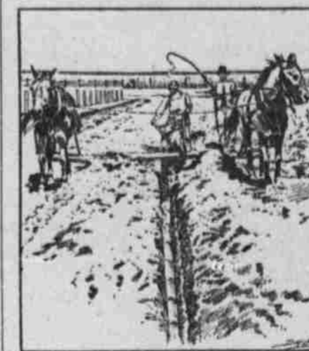
FIG. IX—COVERING THE TILE DITCH.
