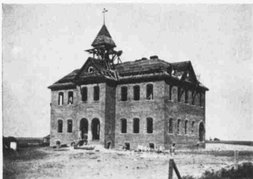
New Emerson School in First Ward.
