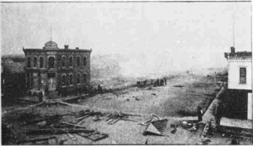
Alliance After the Fire, August 7, 1892.
