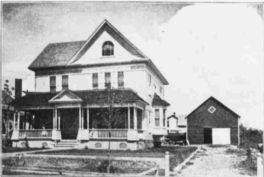
Residence of Geo. W. Clark.
