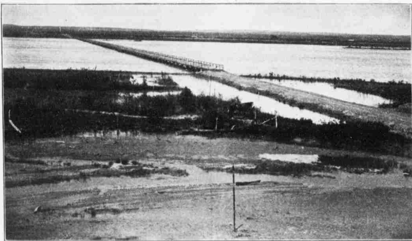
Bridge Across the North Platte River South of Alliance.
