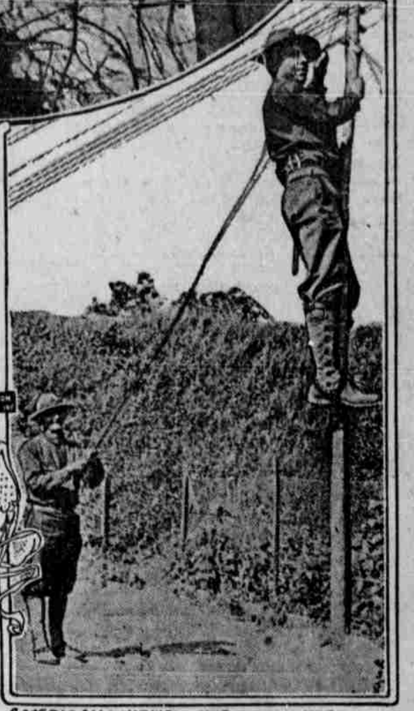
AMERICAN LINEMEN STRINGING WIRES BEHIND LINES
