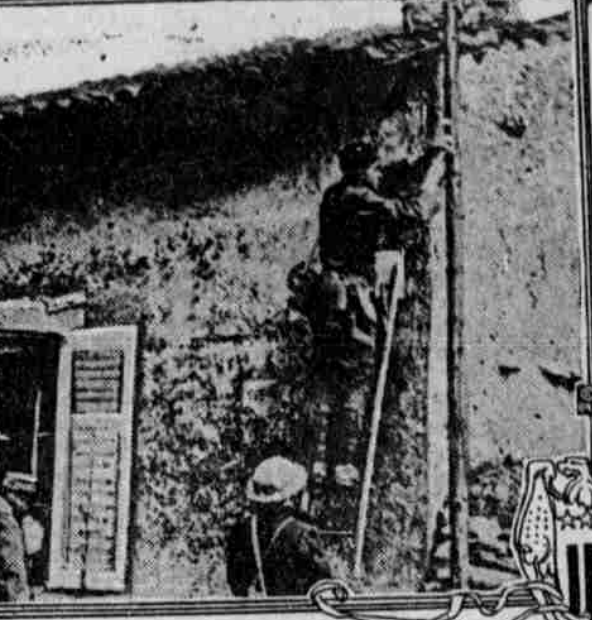
REPAIRING BROKEN LINE "SOMEWHERE IN FRANCE"
