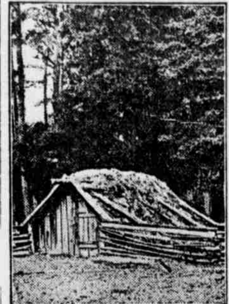
An Outdoor Storage Cellar, Typical of Those Used in the South for Storing Sweet Potatoes and Other Root Crops. It Consists of a Pole and Plank Frame Covered With Sod and Straw.
