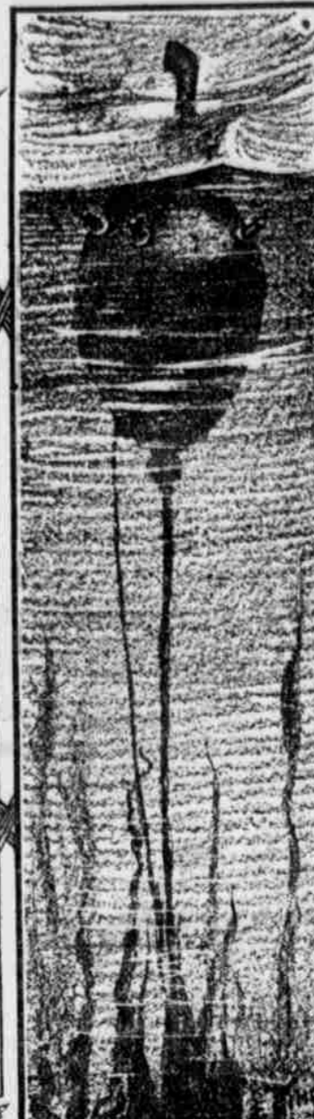
DECOY PERISCOPE ON TOP OF CONTACT MINE
