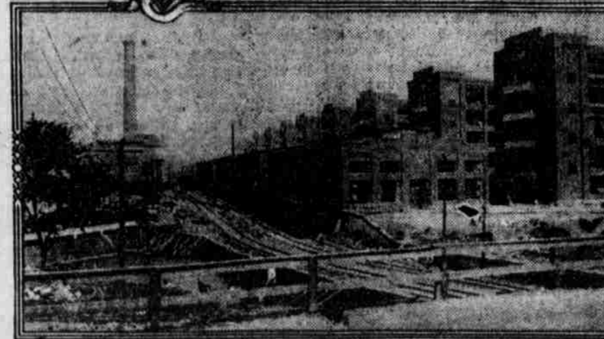
Two Views of Remington Arms Plant (Bridgeport) After Less Than Six Months Construction Work. Ammunition Plant Not Shown.
