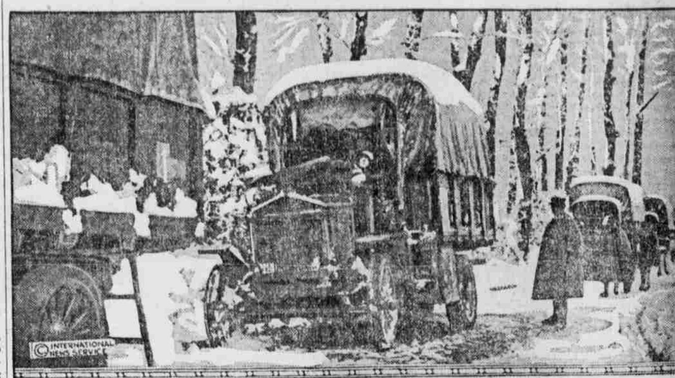
Winter has come again to most of the fighting millions of Europe and their problems are tremendously increased. Transportation becomes especially difficult. The photograph shows part of a long line of motor trucks in France laboring toward the front.
