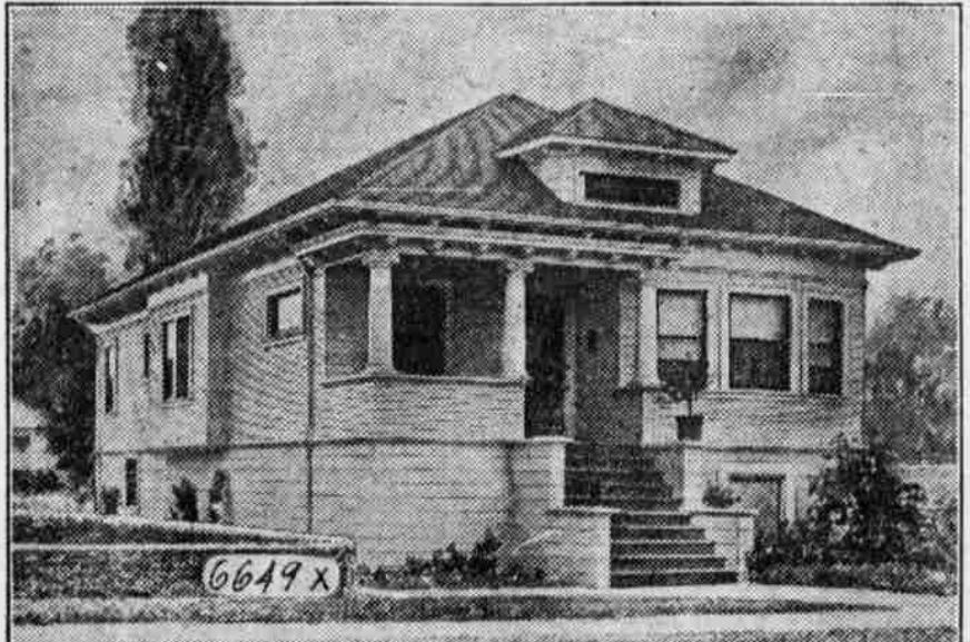
The foundation walls may reach up to the main house floor, or they may stop at or a little above the lot grade line. It may be cheaper to build a superstructure of wood from the ground level up. This is done by placing the sill on the foundation wall, then either build a superstructure of 2 by 6 uprights to support the house sill, or the joists are made long enough to reach from the foundation wall to the plates. With this construction a 2-inch strip is gained into the studding to support the outer ends of the floor joists. The floor joists also are spiked into the studding, so that the building is all tied together at the house floor.
