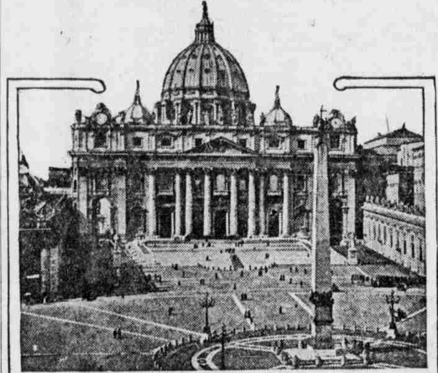
St. Peter's square in Rome was hard hit by the earthquake. The obelisk seen in the foreground in the photograph was shaken and badly damaged; the famous colonnade, seen at the right, was lowered four feet, and an adjacent house, once occupied by the sisters of Pope Pius X, was seriously cracked.
