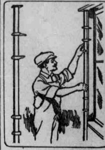
from the top of the door frames, as well as the distance apart. The bar is then placed against the door frame so that the end plate fits snugly at the top, and the markings for the mortise made by drawing lines inside the gauge points.
