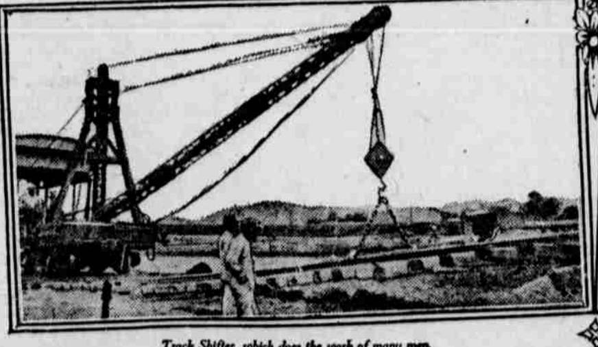
Truck Shifter, which does the work of many men. This device was invented especially for use on the canal work, where frequent shifting of tracks has been necessary.
