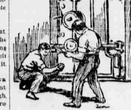
Vault of First National Bank.
