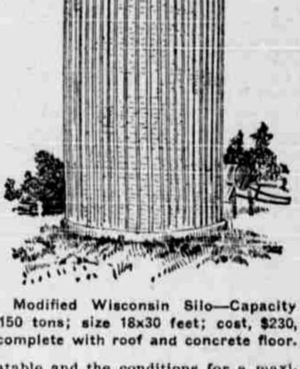
Modified Wisconsin Silo—Capacity 150 tons; size 18x30 feet; cost $230, complete with roof and concrete floor.
