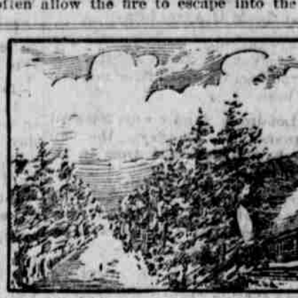
A fire line along a railway with two cleared spaces separated by a double row of trees intended to catch the sparks.
