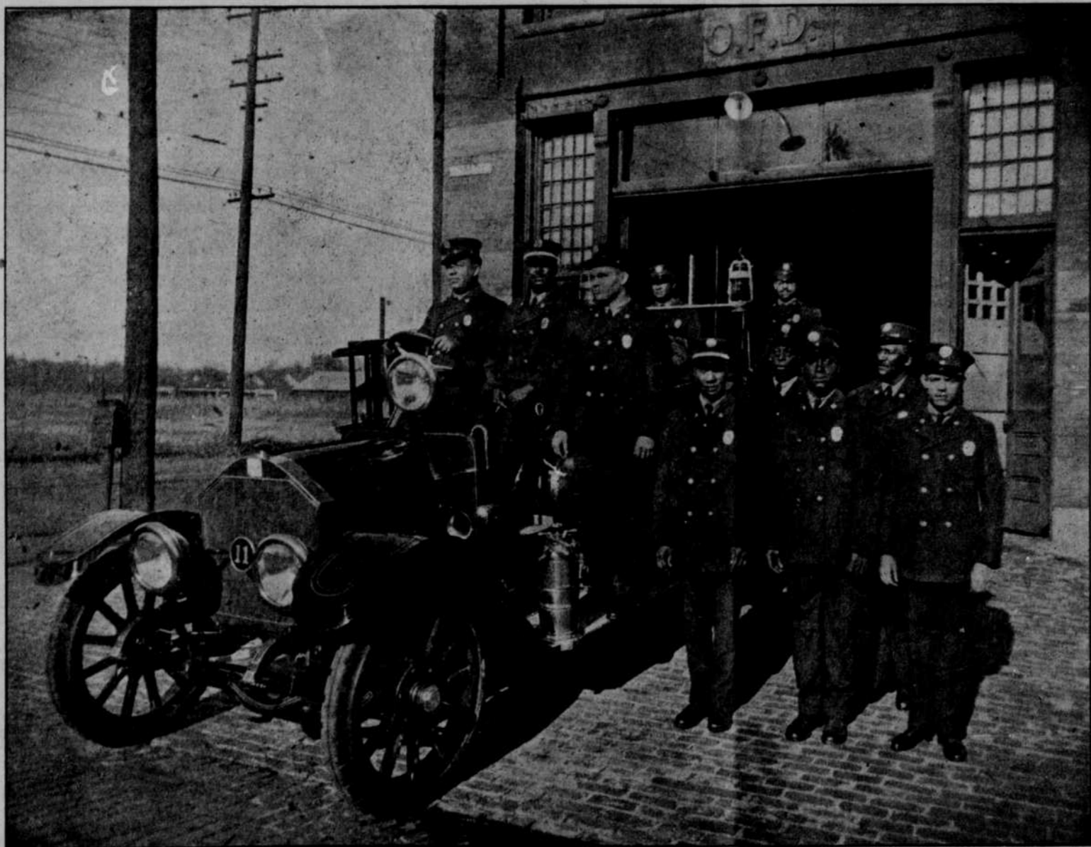
HOSE COMPANY NO. 11 OMAHA FIRE DEPARTMENT
