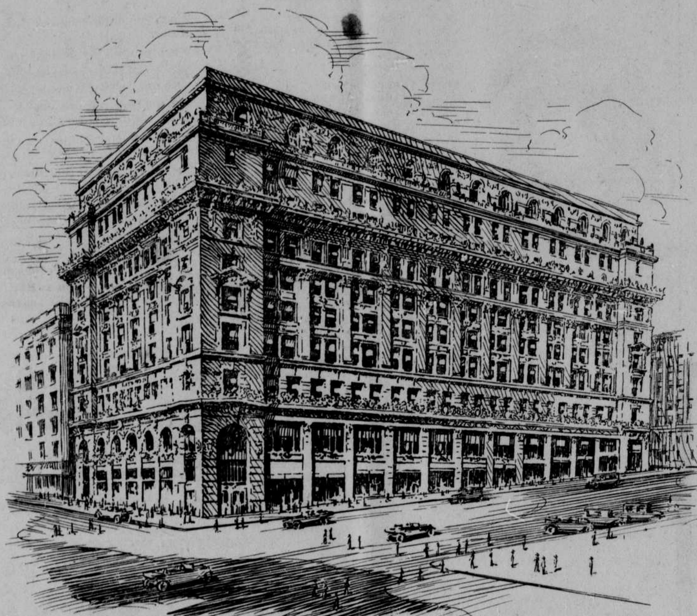
Now a ten-story and basement structure
