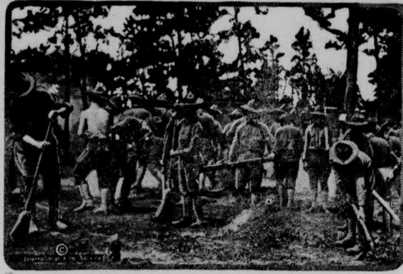
Laying Out the Training Camp Streets.
