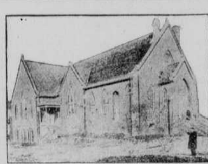
GROVE METHODIST CHURCH 22nd and Seward Sts., Omaha, Neb.
