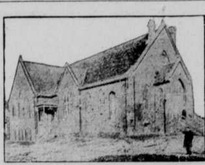
GROVE METHODIST CHURCH 22nd and Seward Sts., Omaha, Neb.
