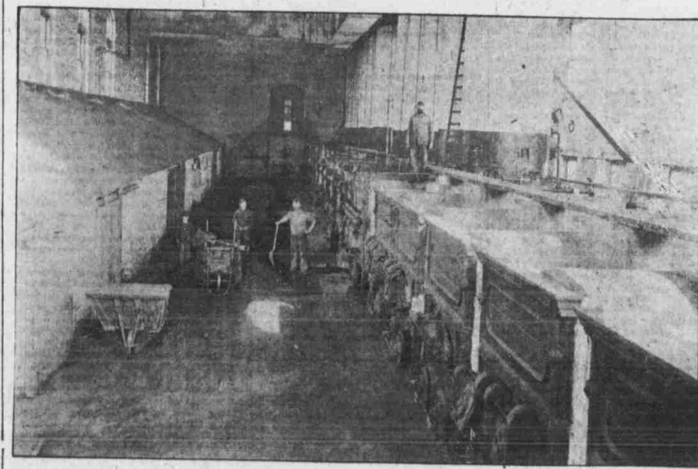
IN THE BOILER ROOM AT THE PUMPING PLANT.
