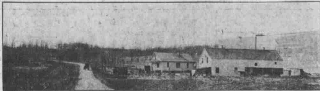
MACADAMIZED ROAD RUNNING THROUGH RALSTON TOWNSITE PROPER, TO BE THE MAIN STREET OF RALSTON.
