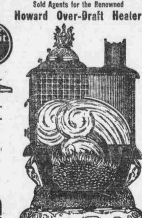
A shovel full of coal will give more heat and lasts longer in a Howard Heater than in any other make. The "Union" has the sole Omaha selling on these marvelous heaters. The above illustration shows the wonderful patented over-draft system used only in the Howard. This system enables this heater to consume ALL the gases and combustible elements in the coal, rendering the stove almost smokeless. Burns every kind of fuel. Many different styles. Easy terms.
