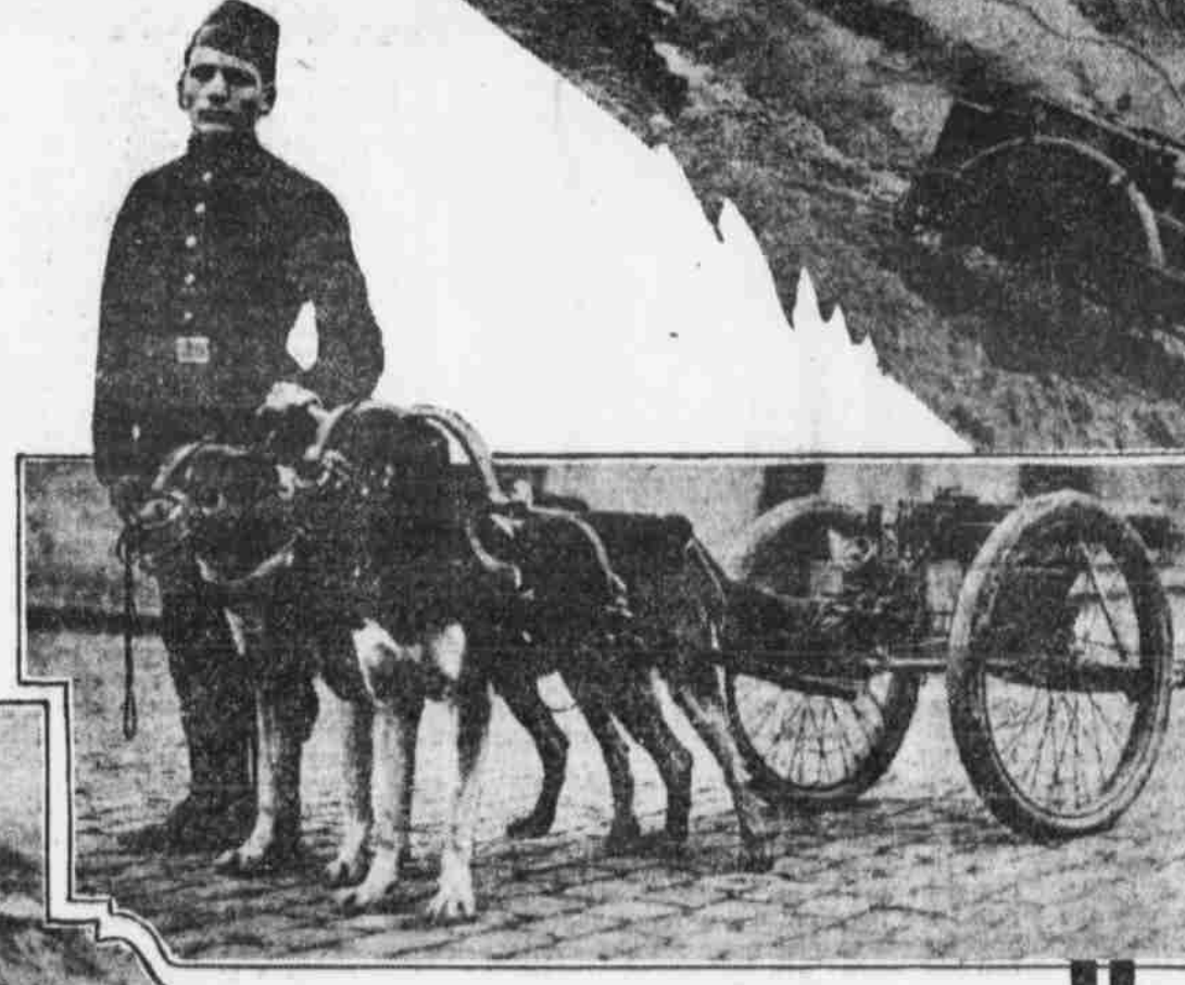
Each Machine Gun on Its Light Carriage of Bicycle Tubing Is Drawn by a Team of Two Dogs, Guided by One of the Gun Crew.
