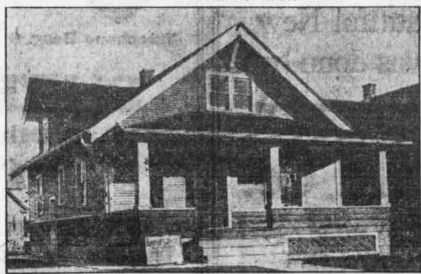
The above plan is from the offices of Everett S. Dodds, architect, and anyone desiring further information relative to the cost of this cottage or the design-
