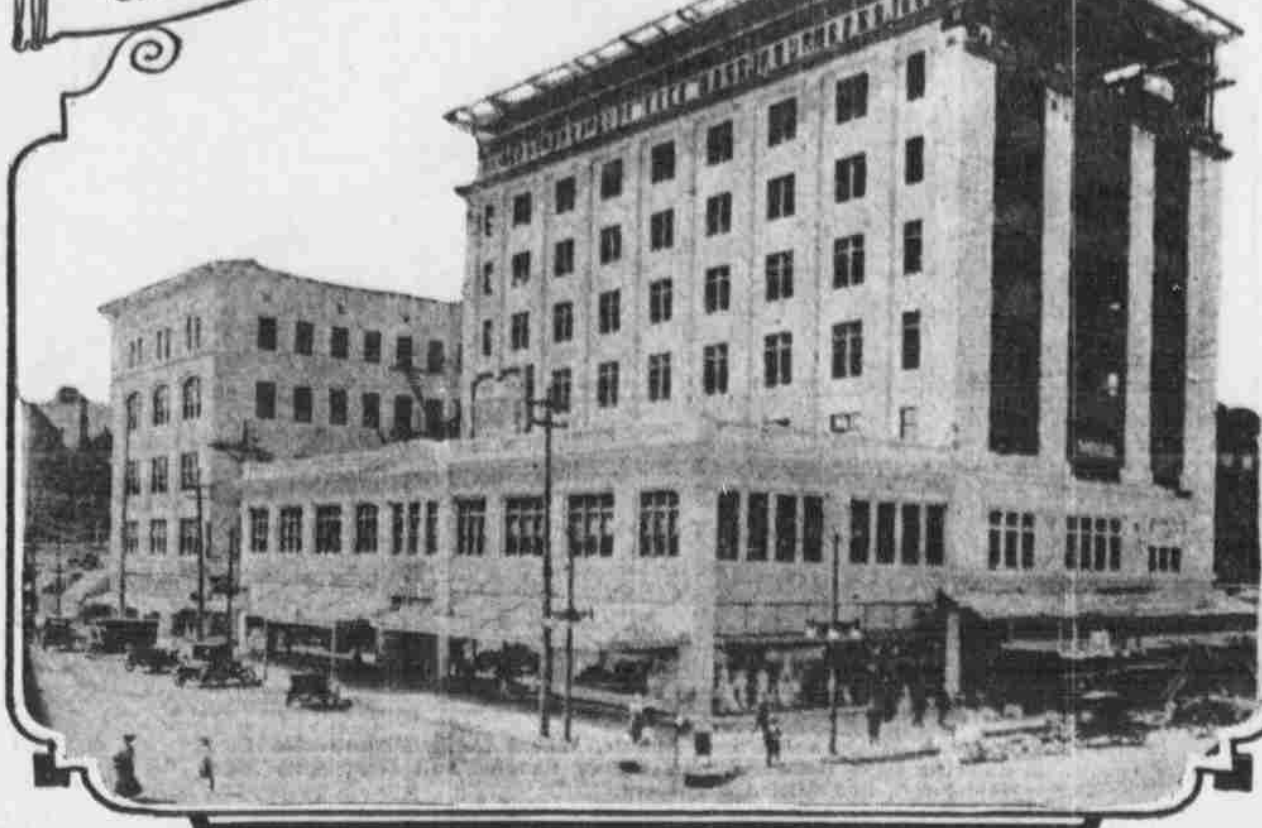
This Building, When Completed, Will Give Lincoln One of the Greatest Department Stores in the State, and Shows How the Business Men of the Community Are Keeping Up with the City's Steady Growth.
