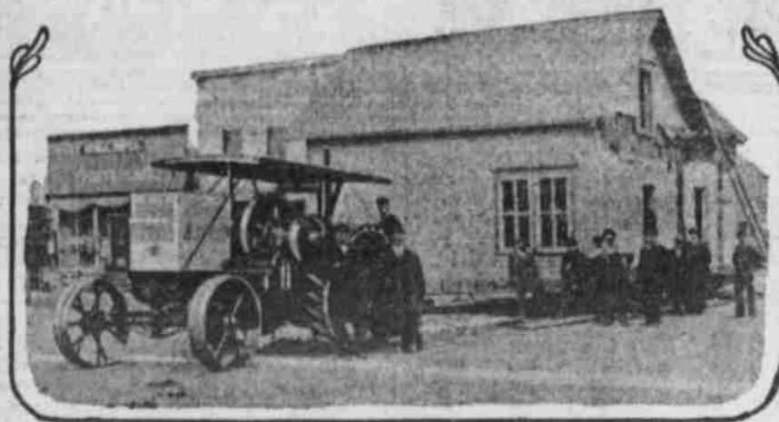
Utilizing a tractor to move a house
