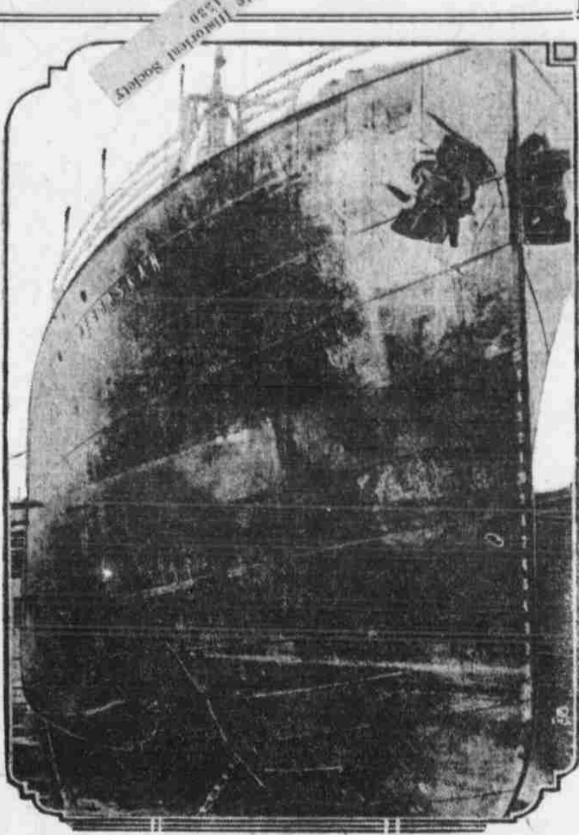
BOW VIEW OF THE NEBRASKAN in dry dock at London, showing immense hole torn in her, presumably by a torpedo fired from German submarine.
