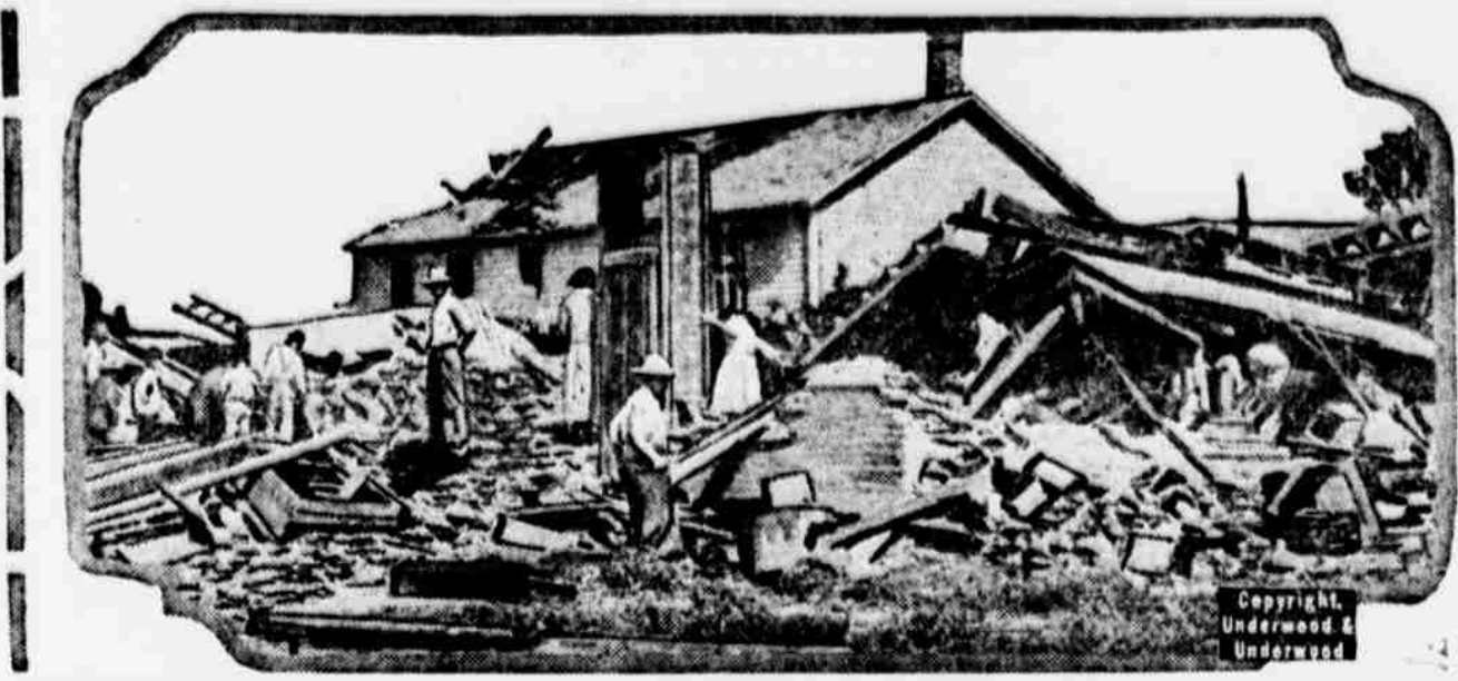
Thirty-five persons were injured seriously by a tornado that swept down on the little town of Leati, Kan., and completely demolished many buildings in the business and residential districts. The photograph shows damage done on one of the residence streets.
