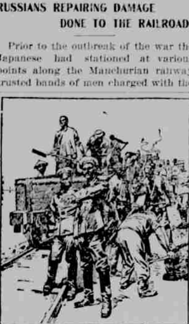
RUSSIANS REPAIRING RAILROAD.
