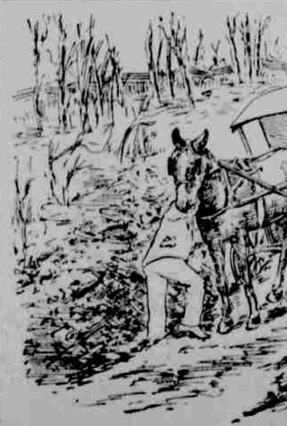
WHEEL-TIRE PHILOSOPHY. —Scene on country road, showing deep ruts and disastrous effects of narrow tires.
