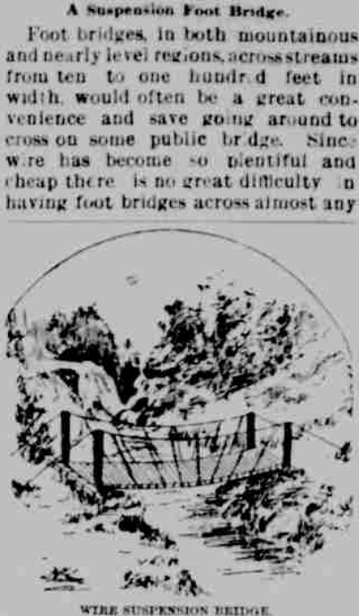
WIRE SUSPENSION BRIDGE.
