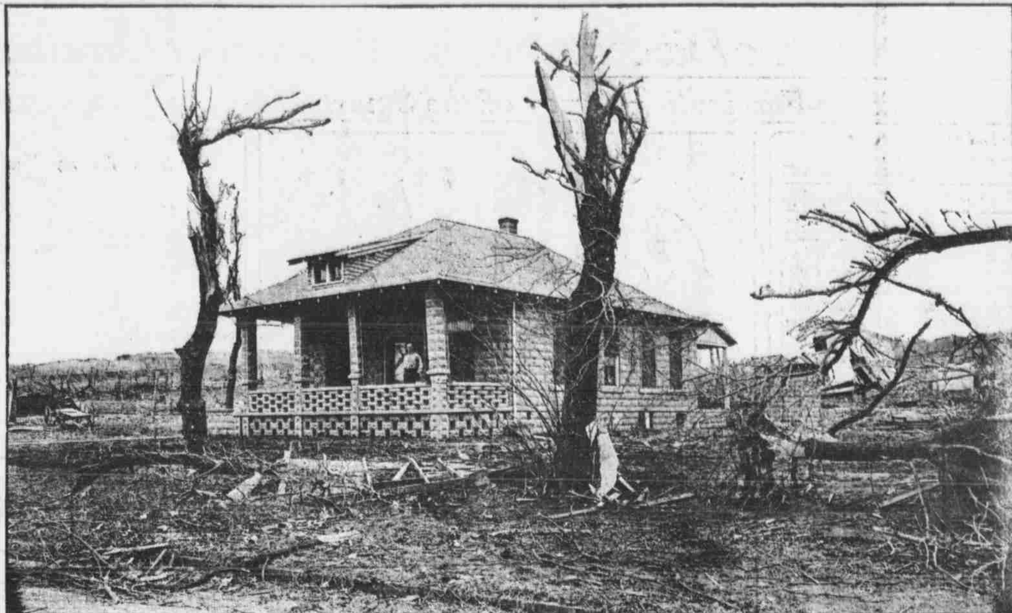
TERRIFIC FORCE OF EASTER STORM IS SHOWN BY DAMAGE DONE TO TREES IN FOREGROUND AND IN BACKGROUND. CONCRETE BLOCK HOUSE WAS NOT INJURED.
