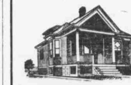
A No. 152 IDEAL Boiler and 265 sq. ft. of 36-inch AMERICAN Radiators, costing the owner $140, were used to heat this cottage. At this price the goods can be bought of any reputable, competent fitter. This did not include cost of labor, pipe valves, freight, etc., which are extra and vary according to climatic and other conditions.
