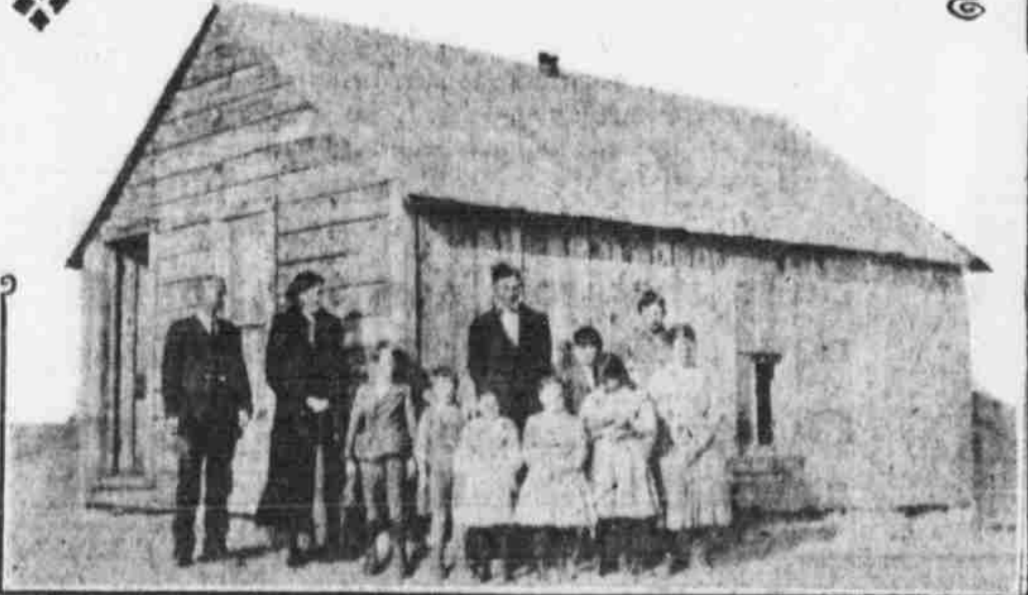
School House District 71 - Chase County
