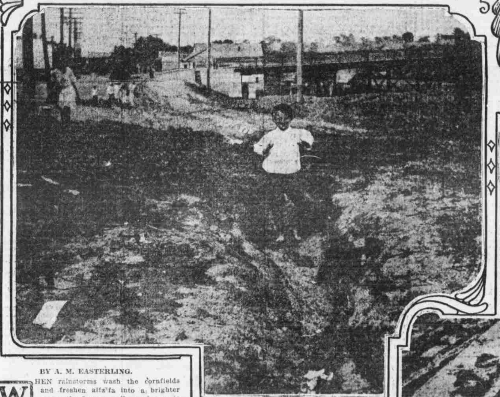
West Entrance to Bancroft Street Viaduct
