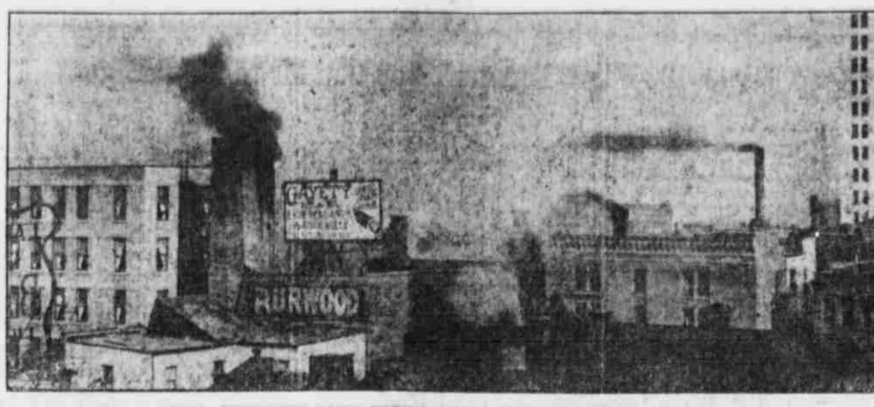
MORE CHIMNEYS POUR FORTH THEIR SOOT AND BLACK SMOKE.
