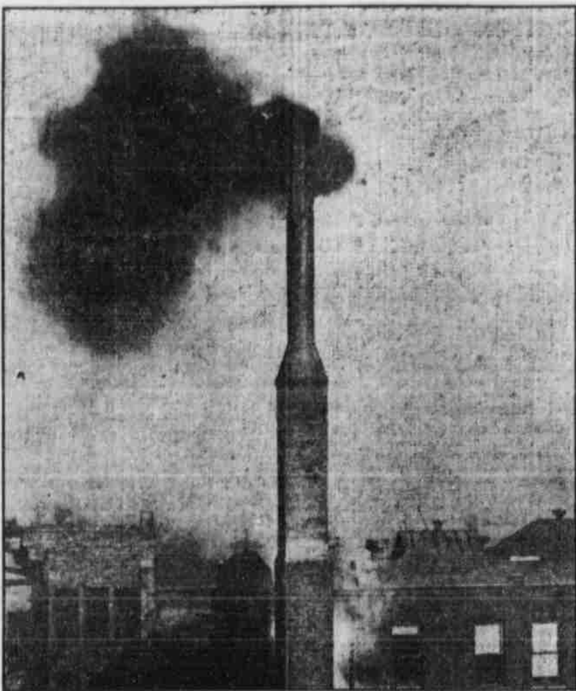
CHIMNEY IN THE REAR OF THE RIVARD HOTEL BLOCK ON PARNAM STREET BETWEEN EIGHTEENTH AND NINETEENTH STREETS.
