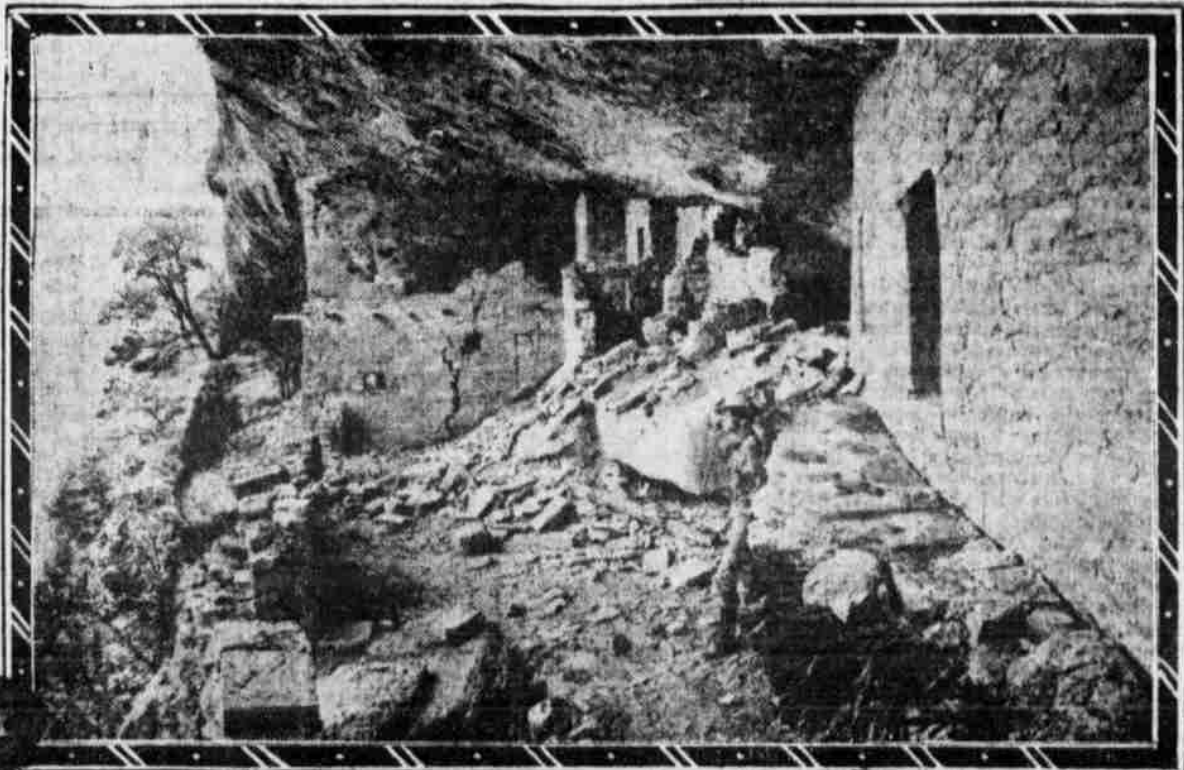
Balcony House, in the Mesa Verde, Colorado, as Restored to Mark the Last Stand of the Old Cliff Dwellers Against Their Enemies from the Plains.
