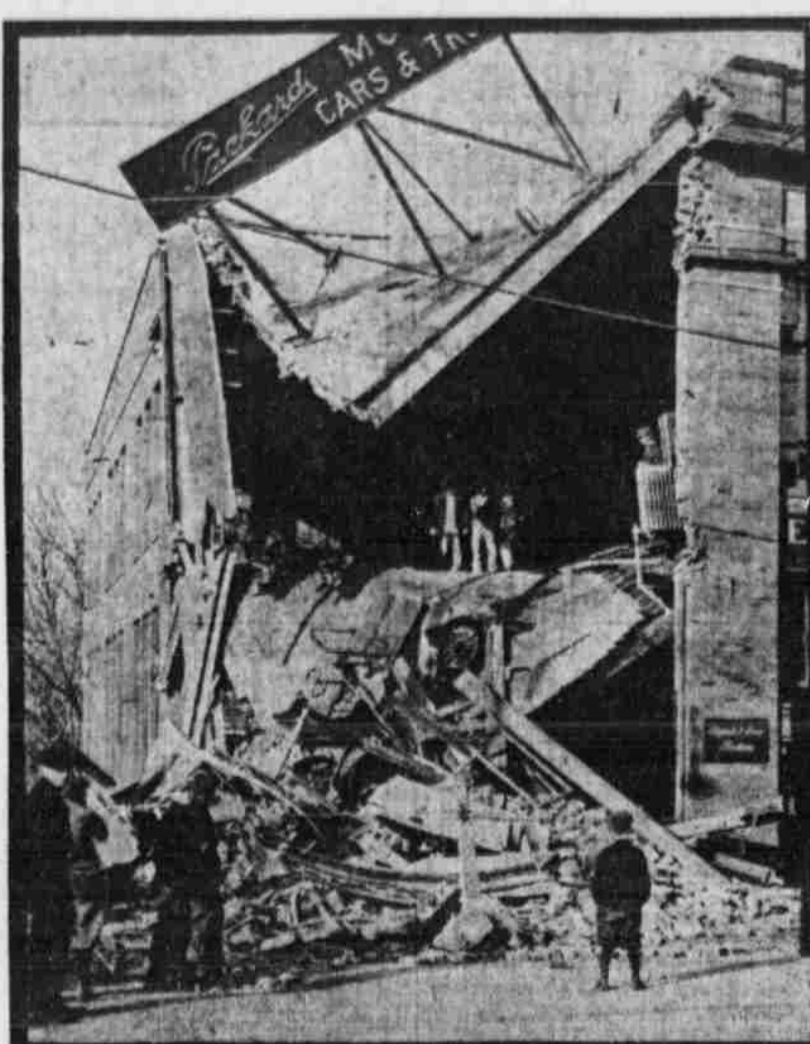
WRECKED BUILDING AT FORTIETH AND FARNAM STREETS WHICH WAS DEMOLISHED BY STREET CAR. —Photo by Bee Staff Artist.
