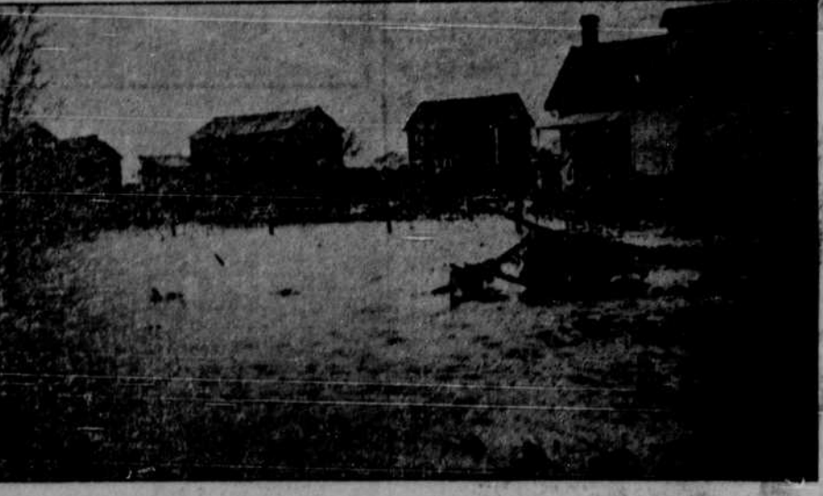
Wm. Schmoldt's home, after the worst was over
