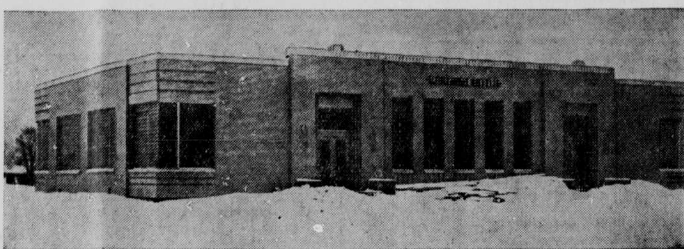
Exterior view of the new Park school in Hibbing, Minn., showing areas of vacuum glass brick replacing the usual windows. This new kind of construction has earned for this novel structure the title of the "Glass" schoolhouse.
